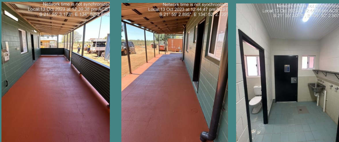
After Laundry & Exterior works completed:
