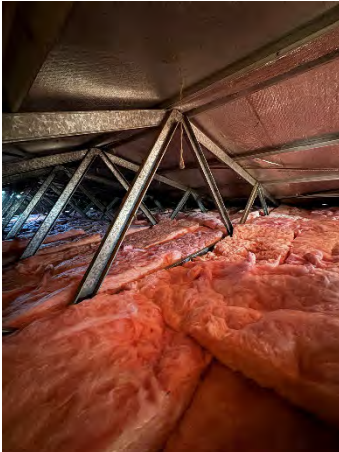
Insulation Installed:
