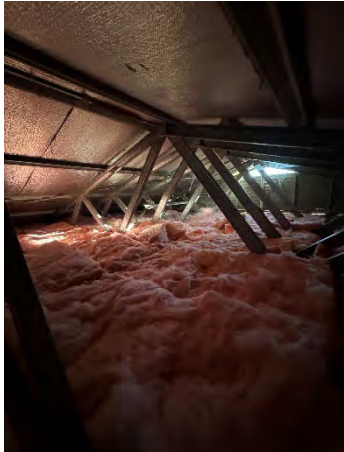
Insulation Installed:
