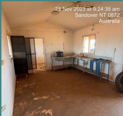
Before works commenced:
