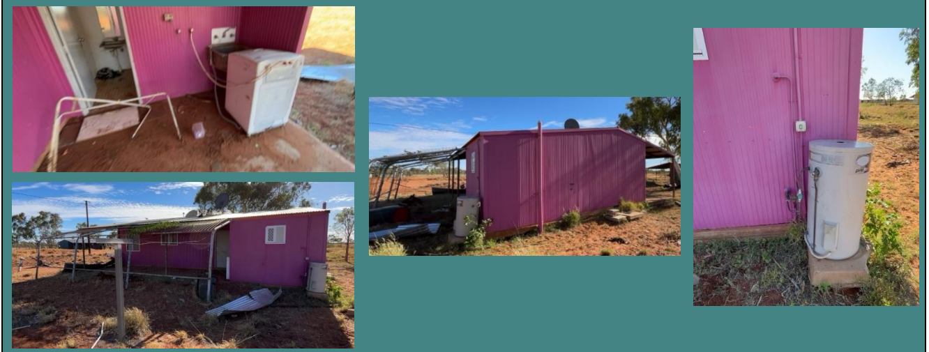
Before Laundry & Exterior works commenced:
