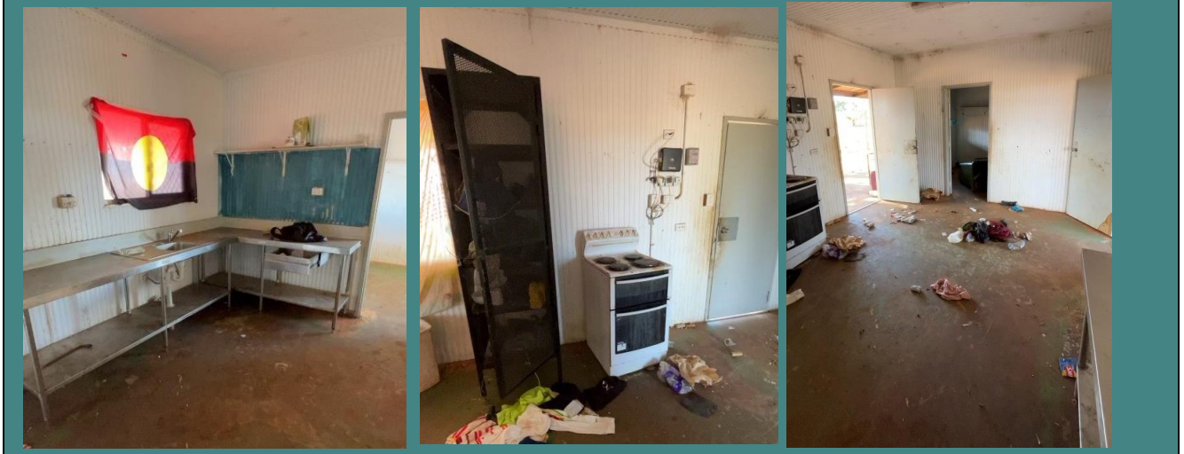
Before works commenced:
