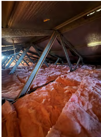
Insulation Installed:
