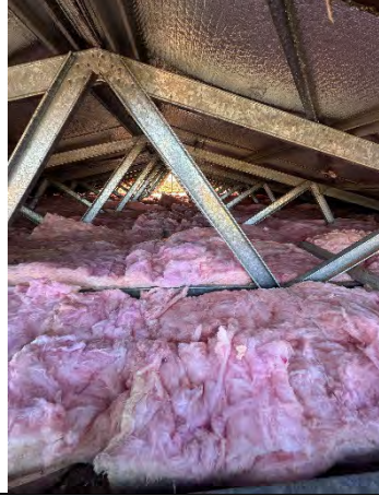
Insulation Installed:
