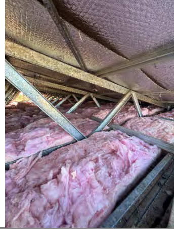
Insulation Installed:
